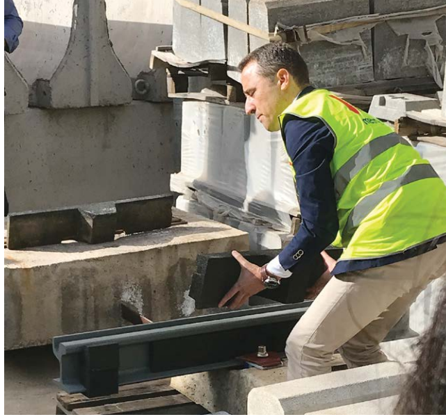
◀ LEFT: Metrotenerife's Project Manager Pablo Oromí showed delegates how the award-winning removable insulating chamber for rail works at the Metrotenerife depot.
