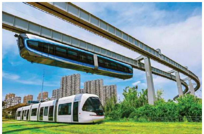
▲ ABOVE: The new monorail crosses over the Wuhan tram line. Optics Valley Skytrain
