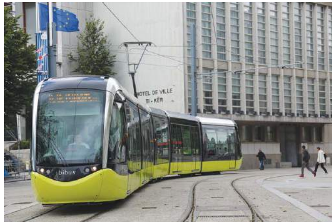
▲ ABOVE: A Brest tram passes the town hall over pointwork already installed for the second line. M. Briand
