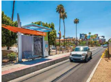
◀ LEFT: Another unusual feature of the Tempe light rail system is that cars are allowed to use the formation - as here at Third Street/Mill. Valley Metro
