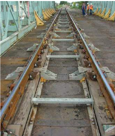
▼ ▲ ABOVE AND BELOW: Beams used in bridging and key blocks and chair used with bullhead rail.
