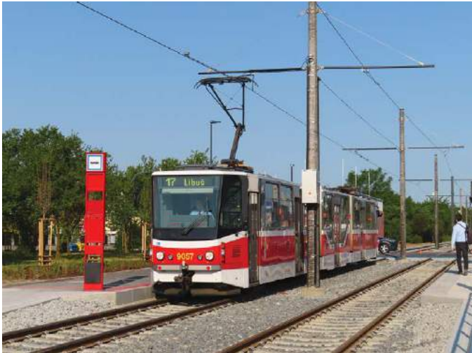
▲ ABOVE: One of the latest extensions to Libuš only took 13 months to deliver - construction started in April 2022, with the route opening in May 2023. Filip Jiřík
