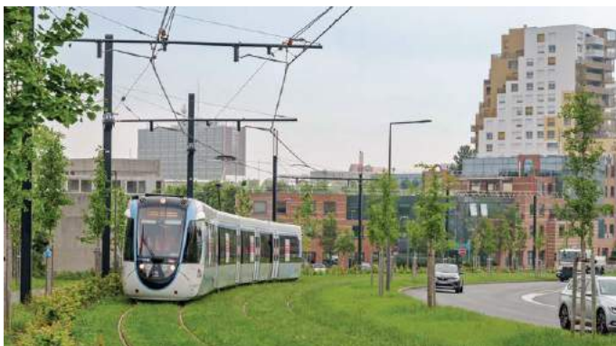
▲ ABOVE: An Alstom Citadis Dualis on the tramway section of line T12. Ile-de-France Mobilités
