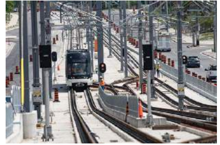
▲ ABOVE: Eglinton Crosstown light rail vehicle testing in Toronto. The new midtown line is scheduled to open this year. Metrolinx
