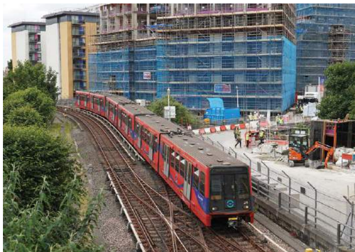
◀ LEFT: Using a new Thames tunnel south of a rebuilt Island Gardens station, the Lewisham route has been a great success. A train led by B90 24 approaches Lewisham terminus, which is sited below the elevated main line platforms, on 9 June 2022. Neil Pulling
