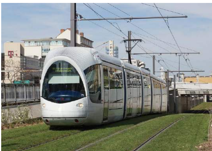
◀ LEFT: While some grassed tram routes still use a concrete bed under the grass, there is only a concrete ladder for support under T10's grass route, which requires less concrete and also means water can drain from the route more easily. On this more traditionally-formed grass trackbed, Lyon Citadis 302 no.872 approaches Lycee Colbert. Neil Pulling
