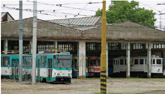
▲ ABOVE: During clearance and rebuilding at Bardejovská depot, a surviving building houses Tatra T6A5 624+625 and works car T3SU 100 . The Ringhoffer DSM 103 white livery was for event promotional use when sited on the otherwise tram-free Hlavná tracks.
