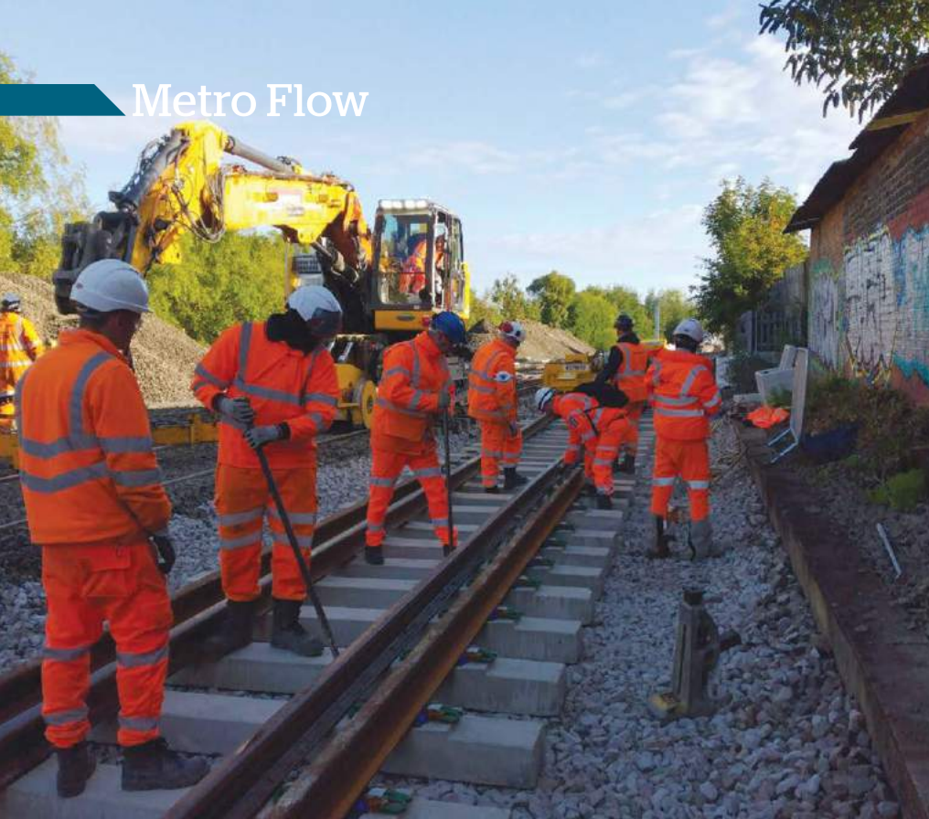
▲ ABOVE: New rail being installed near Ray Roll Underbridge, Hebburn. Nexus
