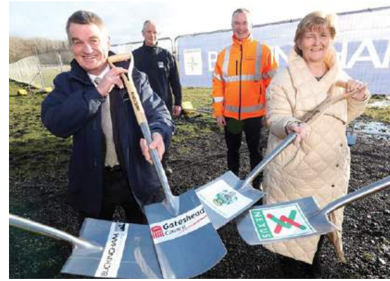
▲ ABOVE: The ground breaking-ceremony for the project took place on 20 January 2021, attended by local officials. Nexus
