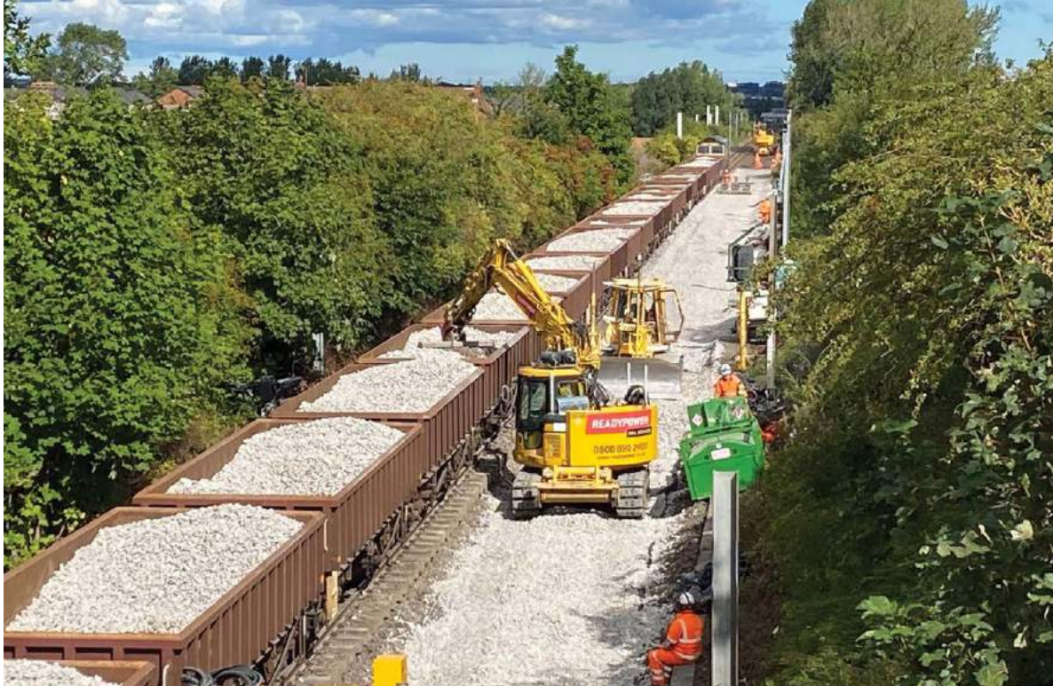
➤ RIGHT: New trackbed installation west of South Drive. Nexus
