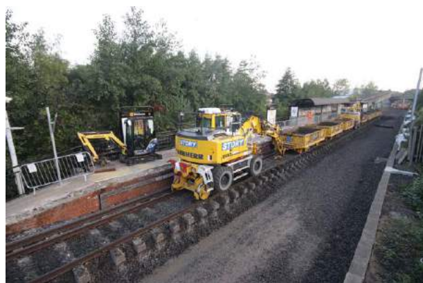
➤ RIGHT: Track lowering at Hebburn Metro station. Nexus
